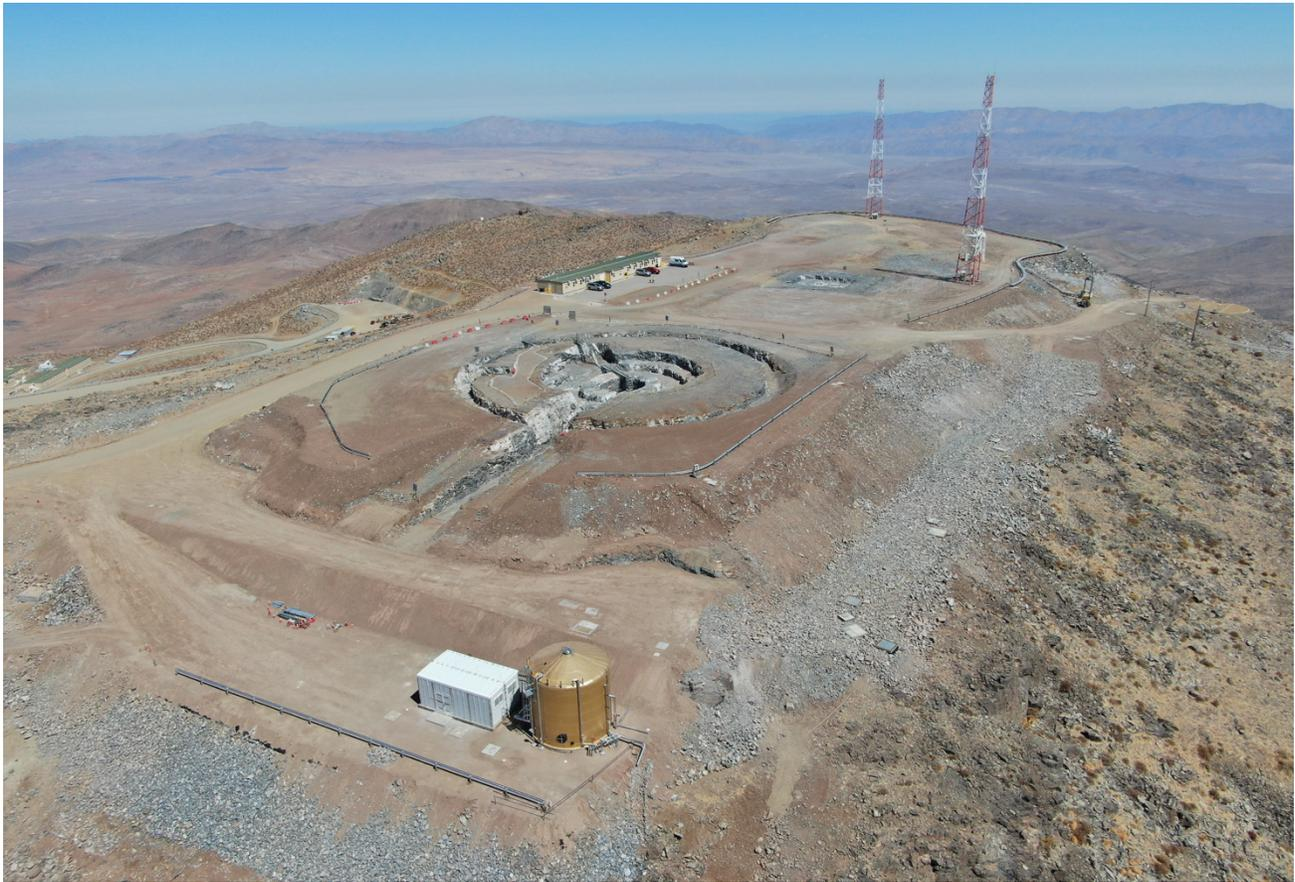
Figure 21. The GMT summit site following completion of the hard rock excavation and utility distribution construction packages.
