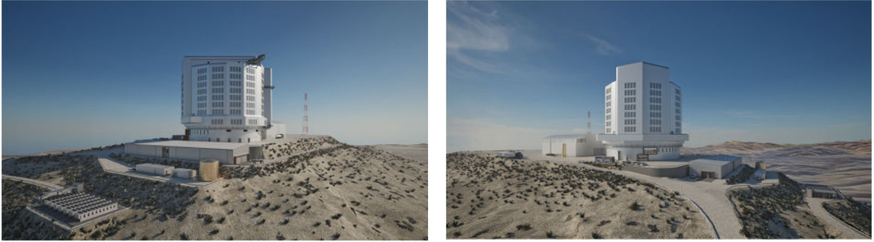
Figure 25. Artist's conceptions of two exterior views of the future GMT Enclosure and summit support facilities. The Summit Support Building housing the M1 washing and coating facilities can be seen behind the Enclosure in the rendering on the left. (Renderings courtesy of IDOM)
