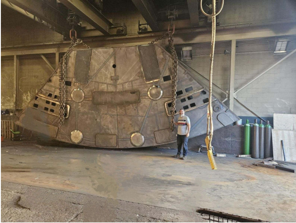
Figure 15. A section of the Azimuth Disk at Dynasty Fab outside Detroit, MI. Once the full Azimuth Disk is completed by Dynasty, it will be shipped to Rockford for integration and testing with the other azimuth structures. (Photo courtesy of Dynasty Fab)
